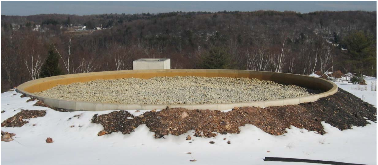
Photo 4. Completed Mitchell Tank. Siphon vault is visible in the background.
