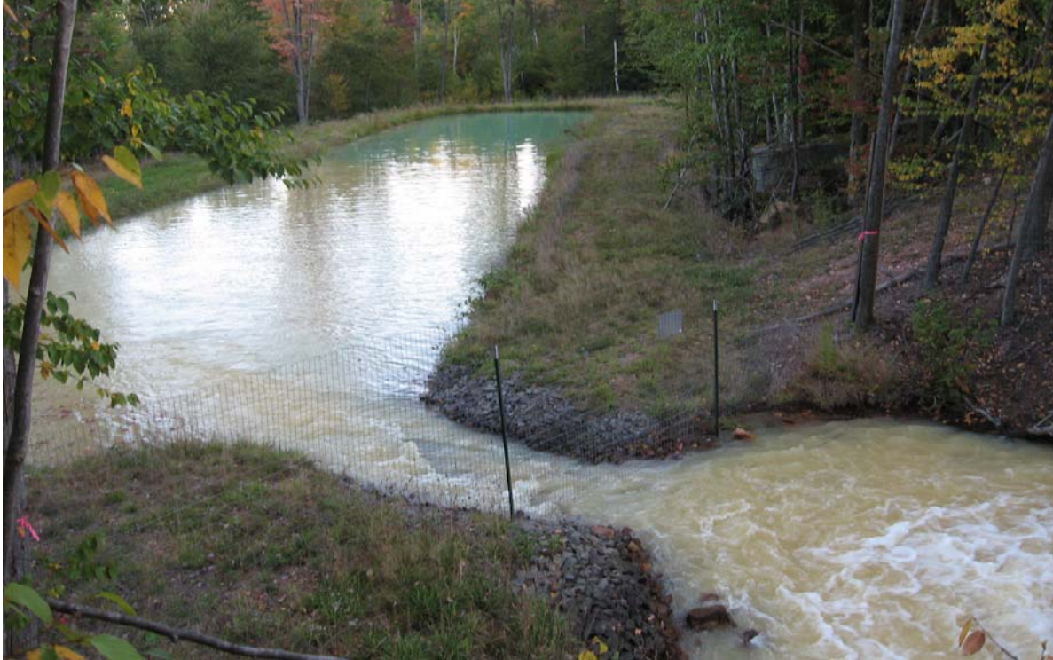
Photo 6. Energy dissipater discharging into settling pond during Mitchell Tank flush.
