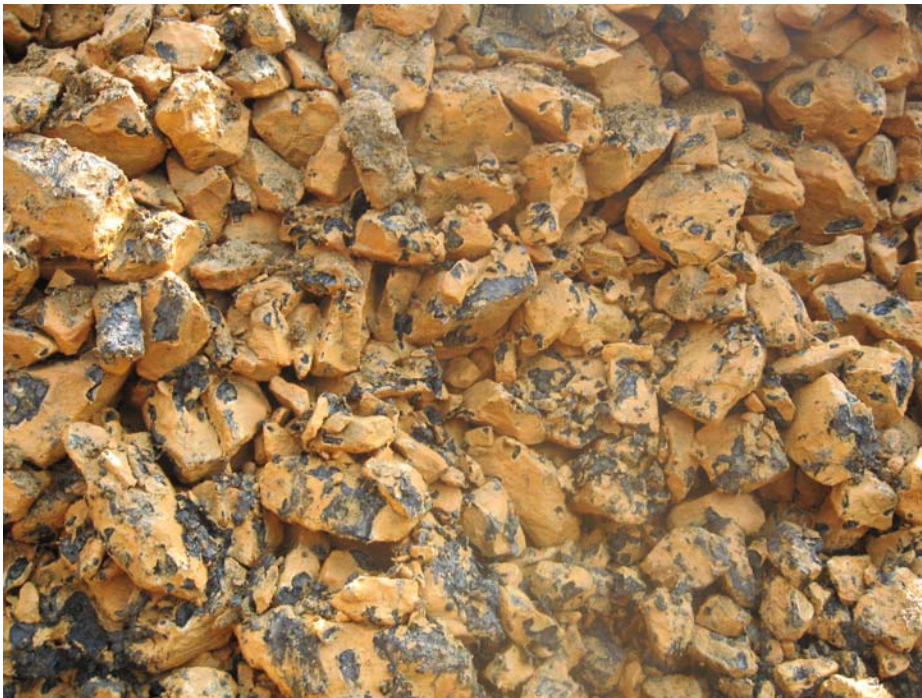
Photo 29. Limestone covered with a scale of metals solids in the Mitchell Tank. The dark patches on the surface of the stone mark contact points with adjacent aggregate particles.
