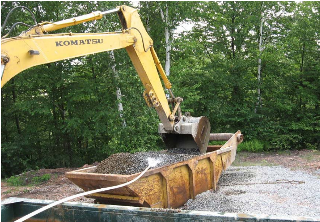
Photo 26. Cleaning of East Box limestone in a stone box. Raw discharge water was used to wash stone.
