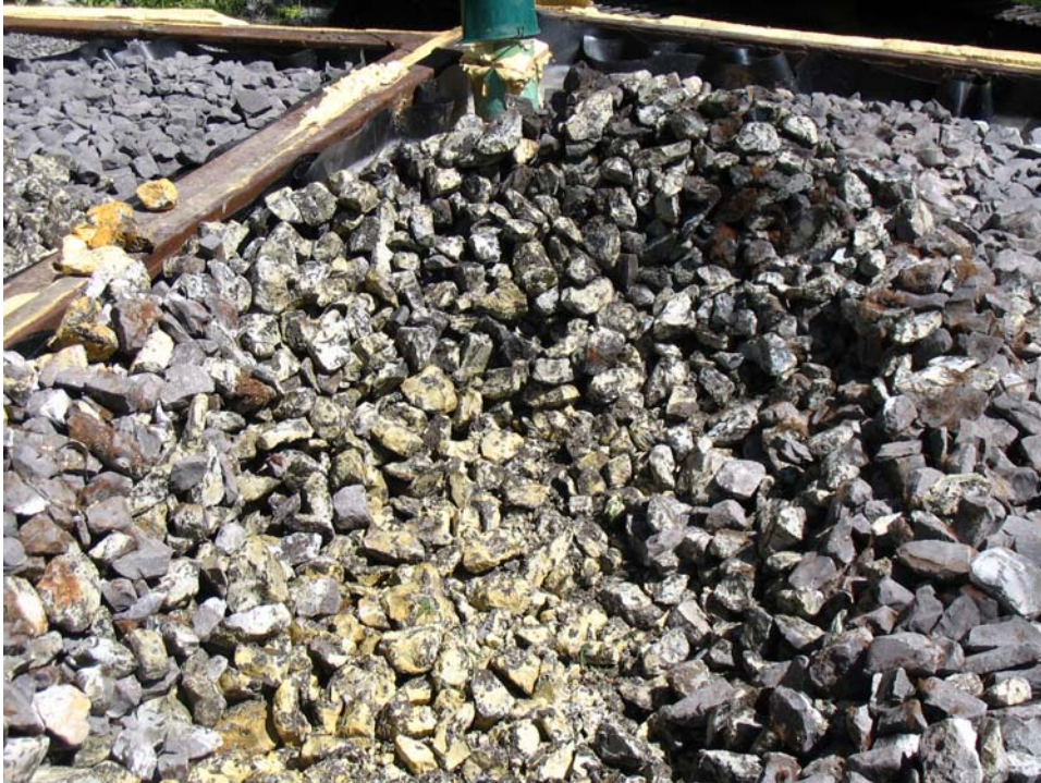
Photo 14. Stone 12 inches below the surface was coated with yellow solids.
