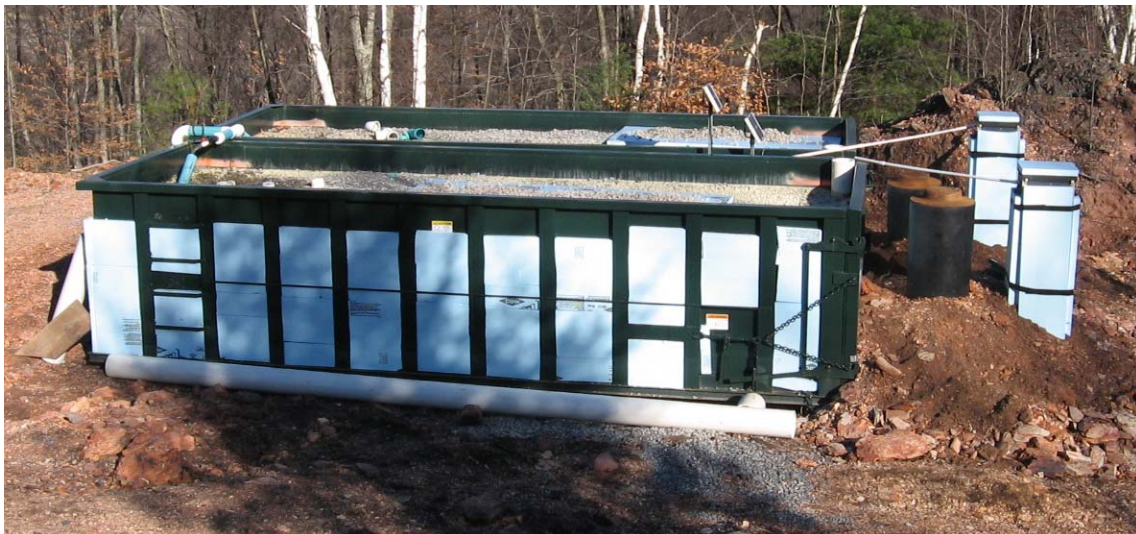
Photo 10. Completed Mitchell Roll Off systems fitted with insulation.
