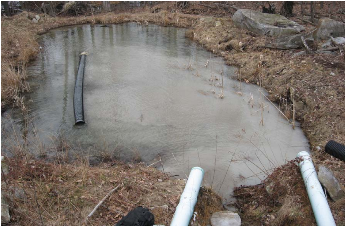
Photo 2. Settling pond that receives effluent from the Jonathan Run systems.
