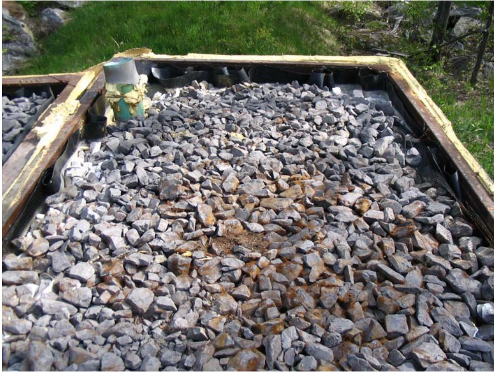
Photo 11. Jon01 box before excavation. Its performance had declined by 75%.
