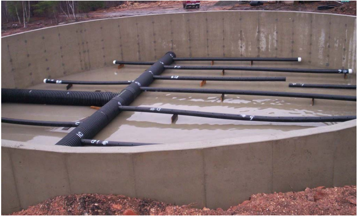
Photo 3. Mitchell Tank under construction with underdrain plumbing exposed.
